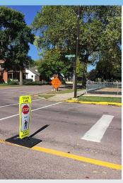
White stop bars are placed in advance of marked, uncontrolled crosswalks at crossing with Rectangular Rapid Flashing Beacons (see page 7).
