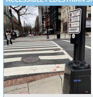
Audible and vibrotactile features that accompany a pedestrian signal head and indicate the walk interval to assist a person who is blind or has low vision in crossing the street.
