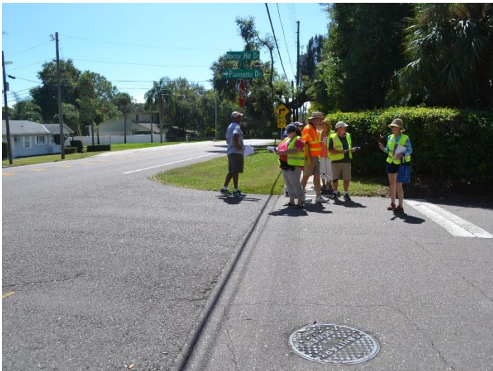
Lack of a marked crosswalk at Palmetto Drive
