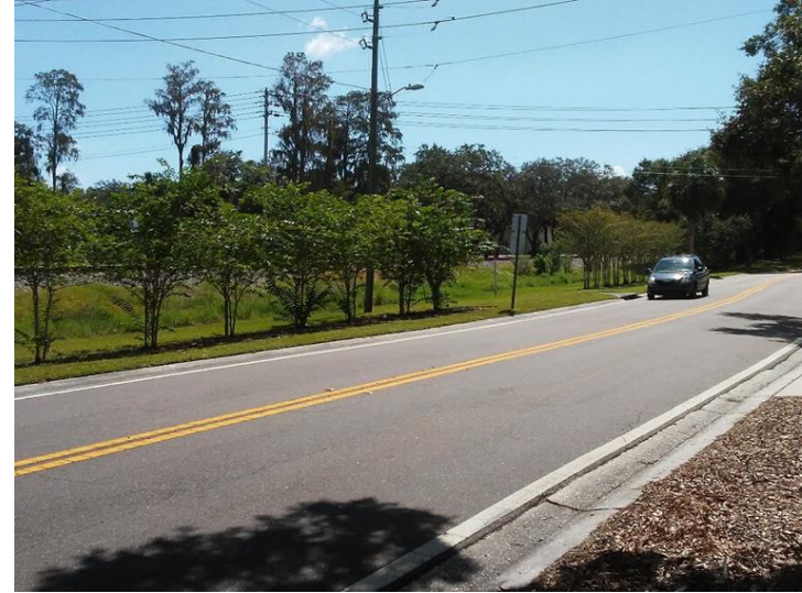
Lack of sidewalks along 9 th Ave. N.
