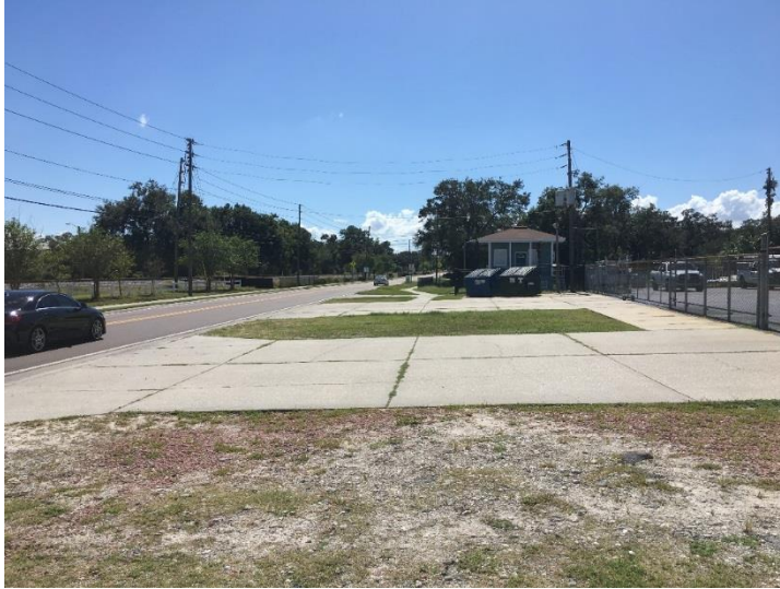
Lack of sidewalks along 9 th Ave. N.
