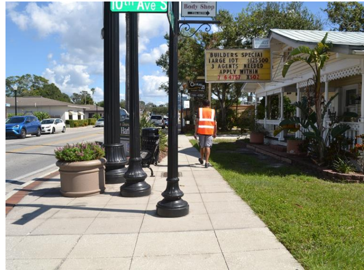
Light pole sidewalk obstruction along Main St.
