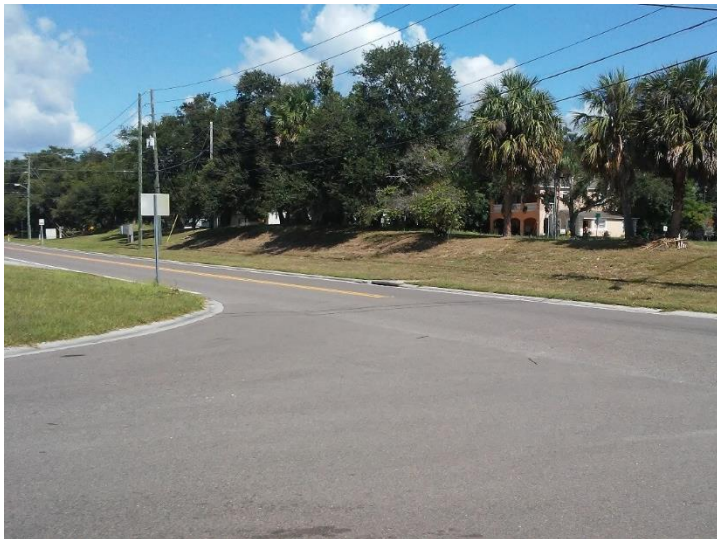
Lack of a marked crosswalk along 9 th Ave. N.
