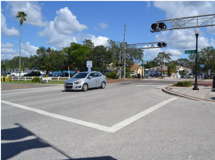
Lack of marked crosswalk along Main St.
