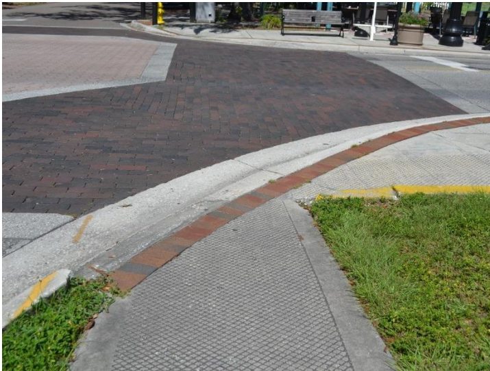
Inadequate sidewalk taper along Main St.
