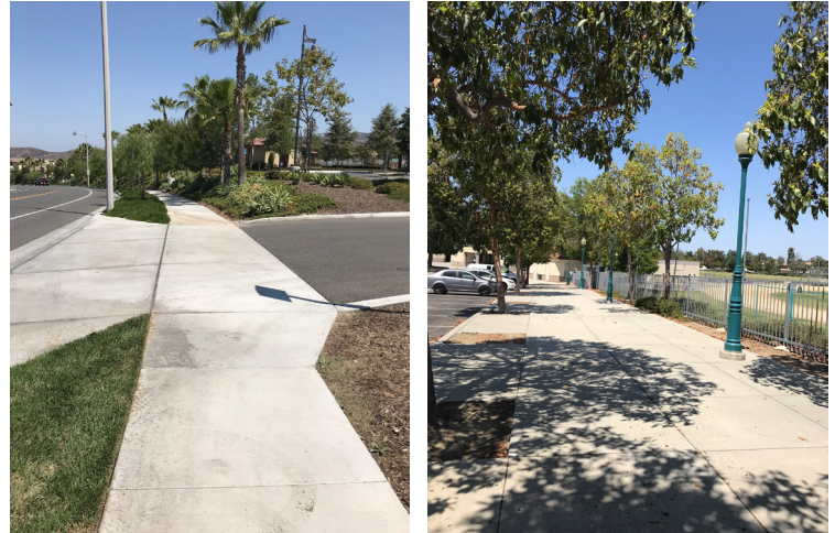
Left: Level walking path provides a continuous walkway across a driveway. Right: Trees improve the attractiveness of the walking path, and pedestrian-oriented lighting ensures visibility for people walking in early or later hours.
