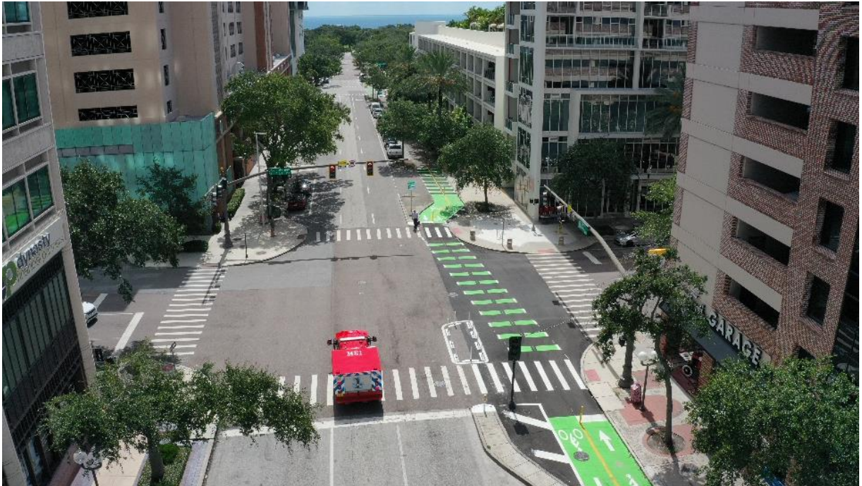
After intersection improvements including interim “wedge” island
