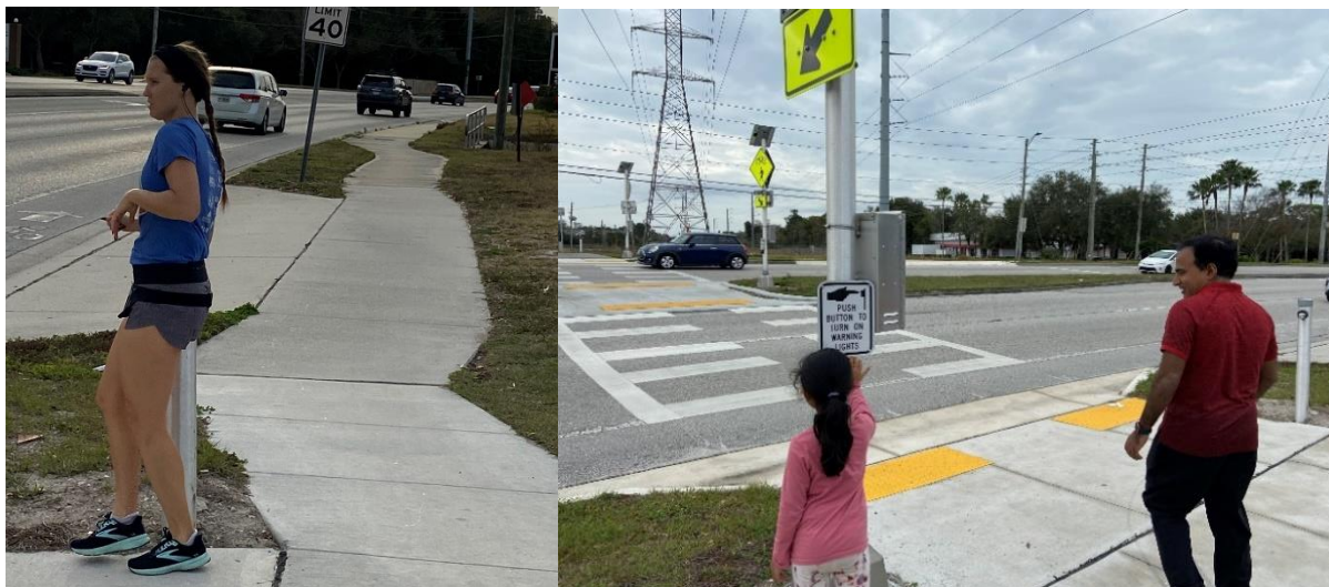
Additional RRFB Activation Pole – A Second Pole Added to Improve Access
