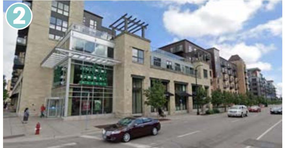
2 Neighborhood supporting grocery store with multi-family residential above and a shared parking garage for businesses and Park and Ride service
