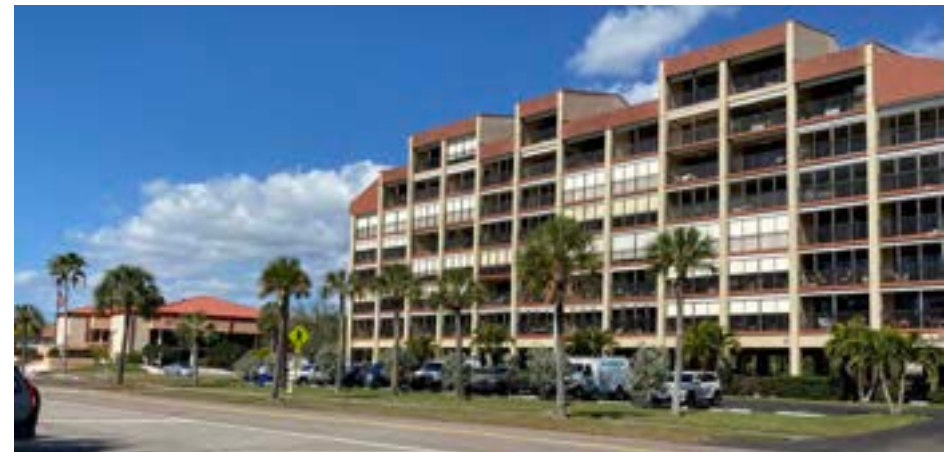
Multi-family housing along Sunset Drive S
