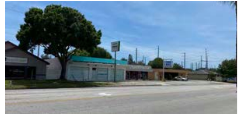
There are many one-story commercial buildings, some vacant, along Central Avenue.
