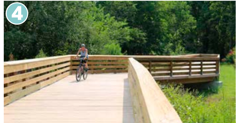
Multi-use trail that extends from Bear Creek Park into the southern neighborhoods
