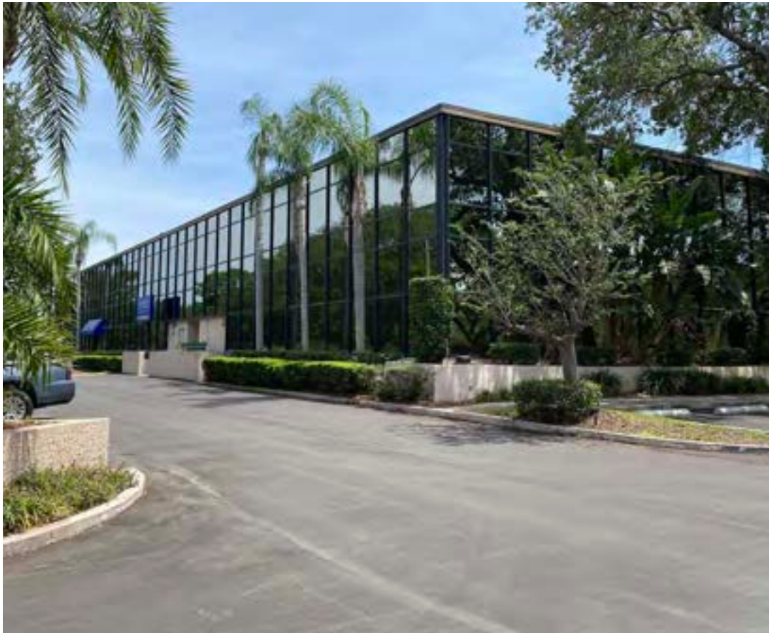
Large office and employment centers located near the SunRunner stations
