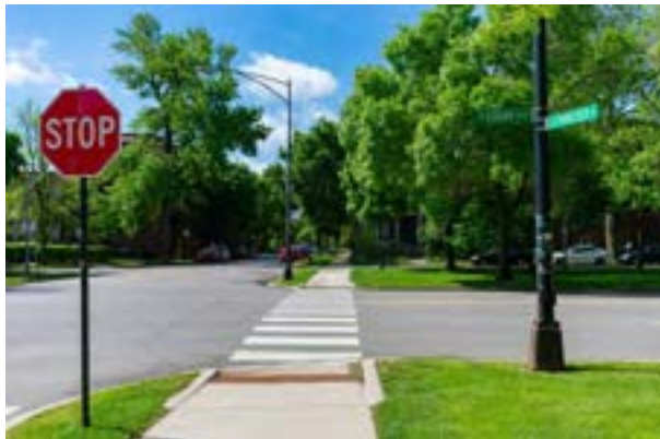
High visibility crosswalk with ADA-compliant curb ramp
