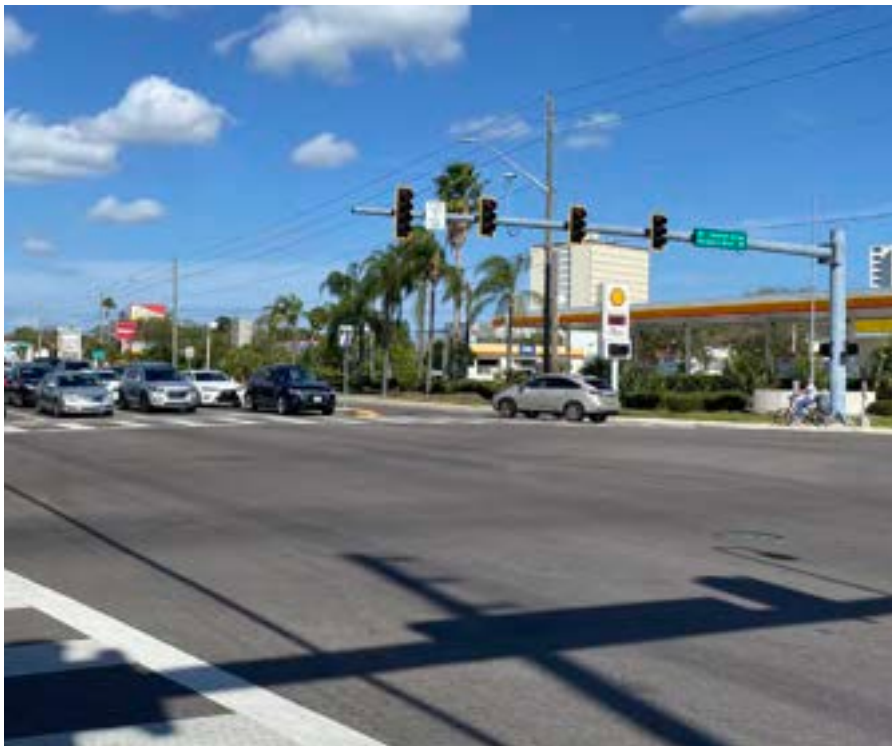
Intersection at Pasadena Avenue S and Sunset Drive S/Gulfport Boulevard S
