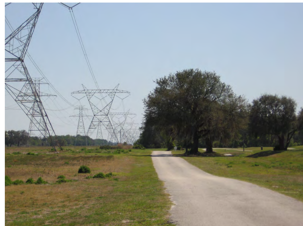
3 An existing Fox Hollow Golf Club service road located within the Duke Energy corridor.
