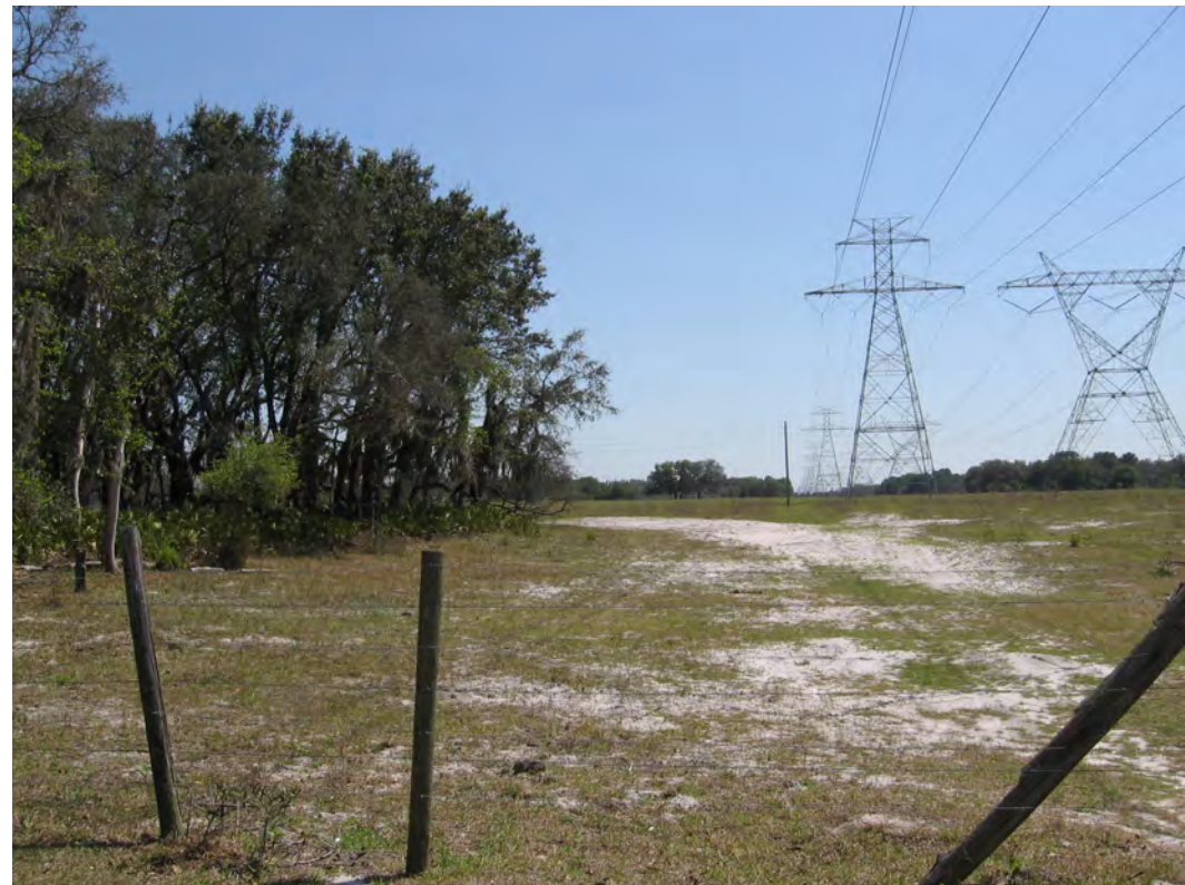
4 View looking south along the Duke Energy corridor at the Pasco County line.
