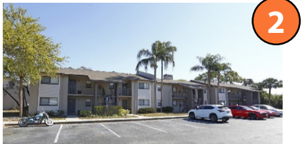
Reserve at Clearwater - 6550 150th Ave N, Clearwater, FL 33760
