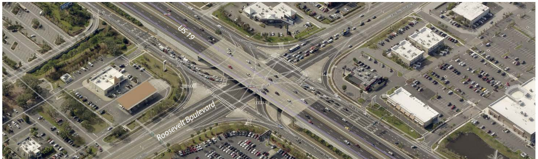
Figure 18. Existing Conditions at US 19 and Roosevelt Boulevard
